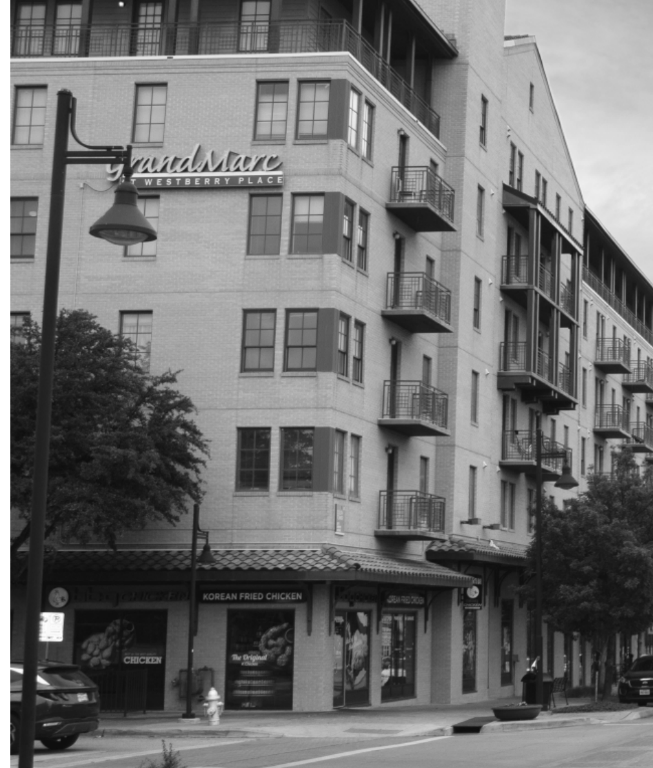
Berry Street view east
